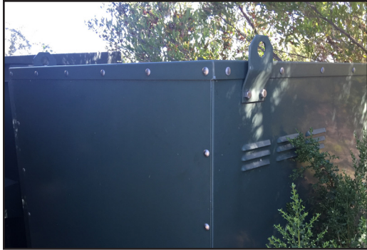
15kV Single Way Switch
