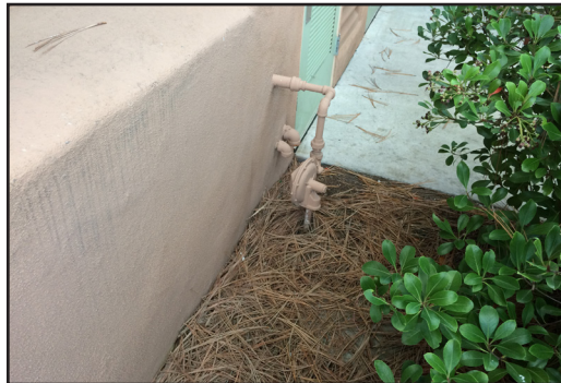
Building 600 - Gas supply into building with gas pressure regulator along building exterior.
